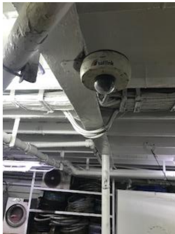
Figure 9: Photo of the camera installed on board the vessel in the brailer room to monitor the individuals that are brought on board the vessel
