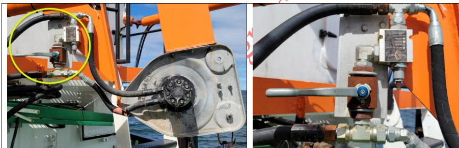
Figure 3: The hydraulic by-pass valve (Limiter) at left of the hauler wheel
