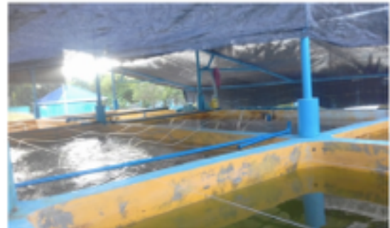
Figure 12. Concrete 9-ton tanks for the culture of tilapia and chlorinated water
