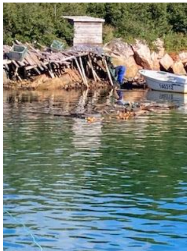
Figure 11: Gear being hooked near a collapsed wharf in Occasional Harbour
