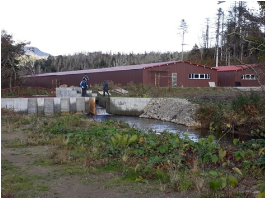
Figure 5. Workshops and fish ladder
