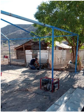
4.- Painting of structure to prevent corrosion
