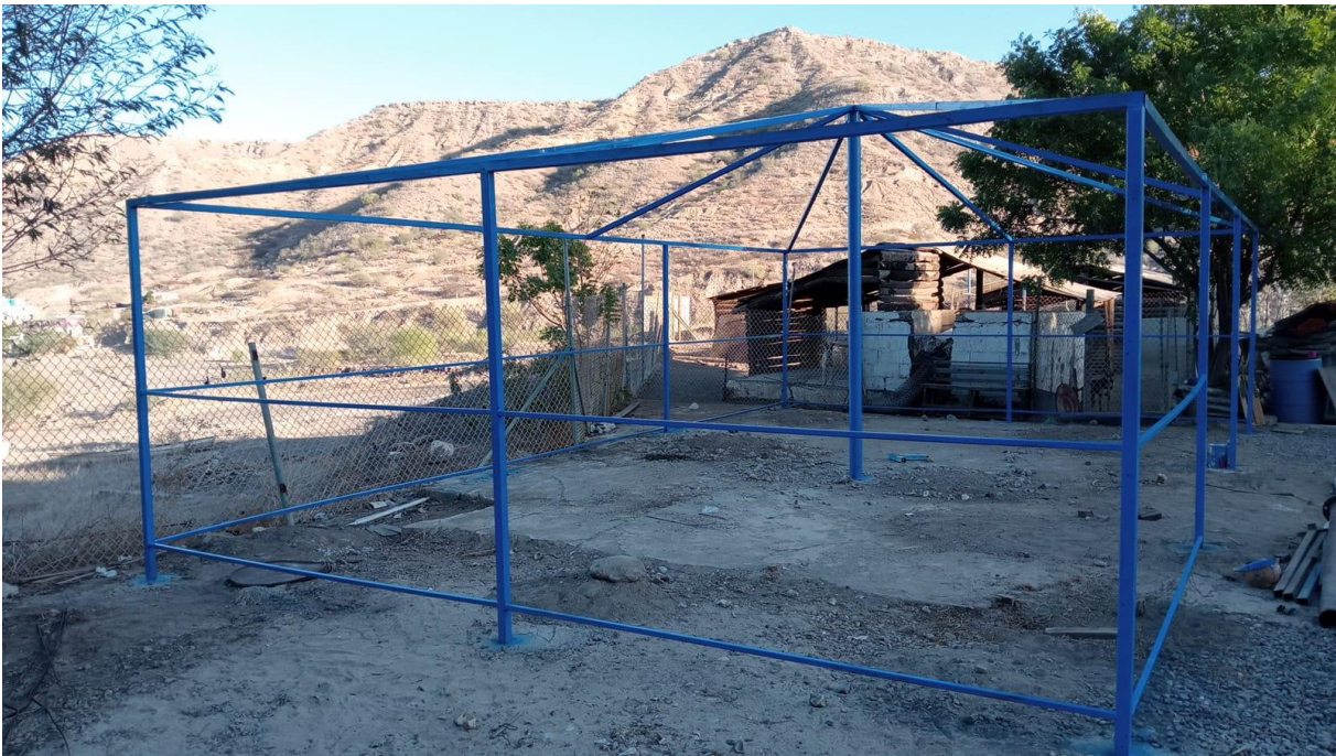
4.- Painting of structure to prevent corrosion
